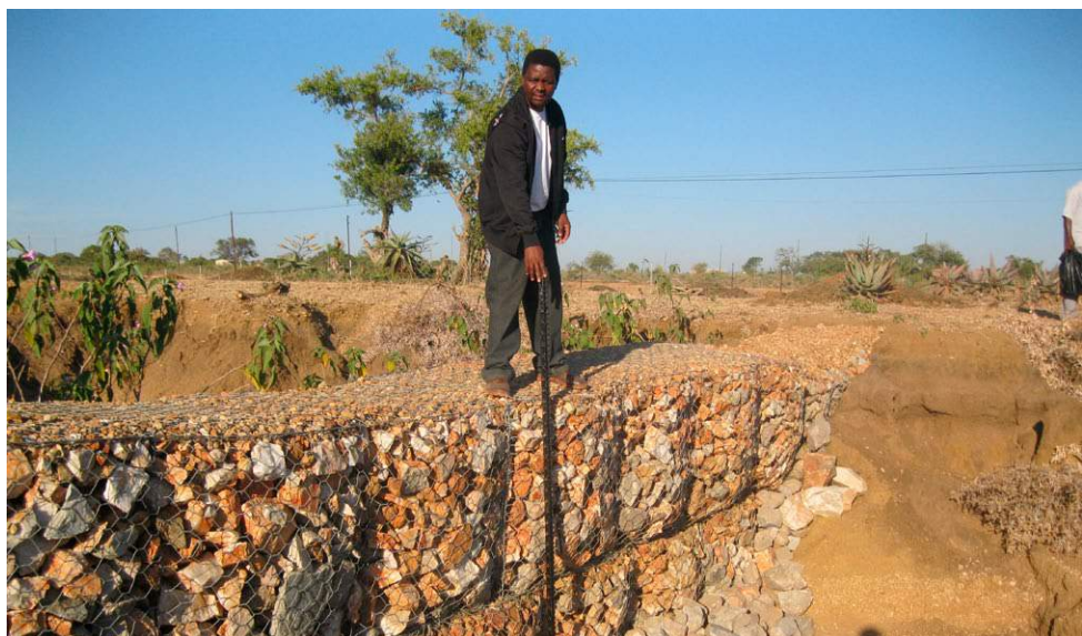
Local people built stone walls using gabion cages, which help to stop erosion
